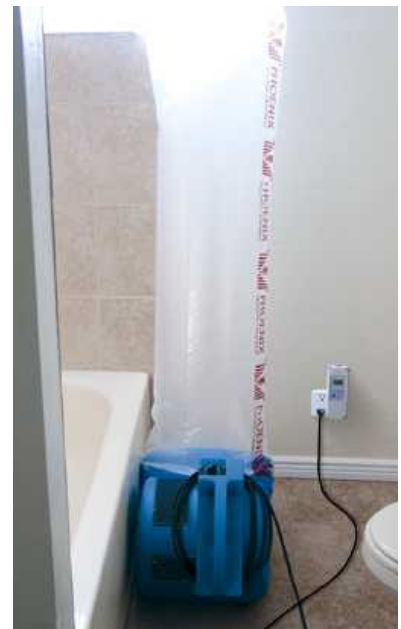
Air mover with ducting connected to Exhaust Controller
